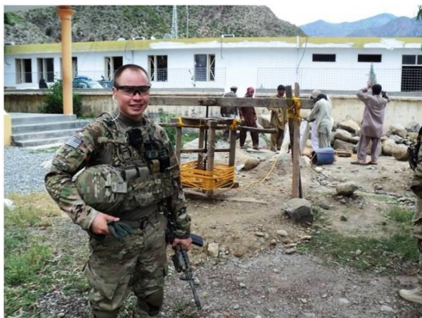
1LT Antioho stands near Afghan construction workers hard at work.
