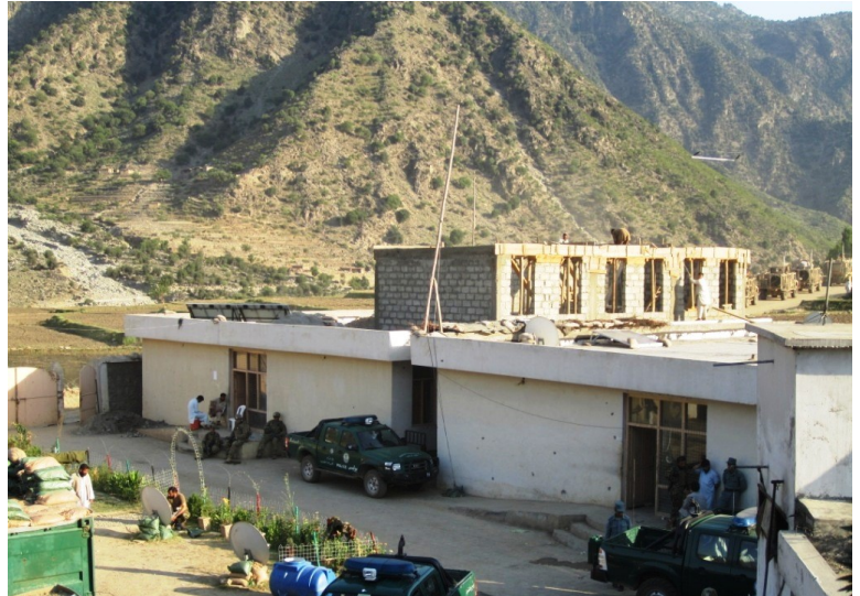
A new meeting room at the District Center that A CO helped build.
